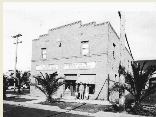
2 The Anderson Building was built in 1927 by George and Lillie (Brown) Anderson. They added the 2nd story in 1928. It housed the post office (Lillie was postmaster, a drygoods store, and an early telephone exchange. Note the large cable on the upper right side.
