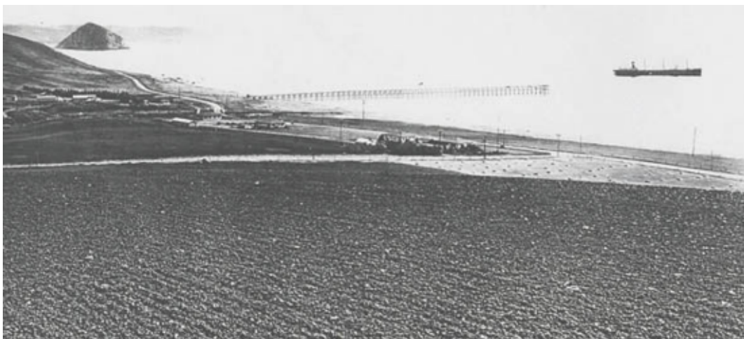
Figure 1: Early on in Standard Oil's use of Estero Bay for loading oil tankers, this steel pier was used for docking them and pipelines ran the length of it. It was deconstructed in the 1980s after being replaced by underwater pipelines years before.
