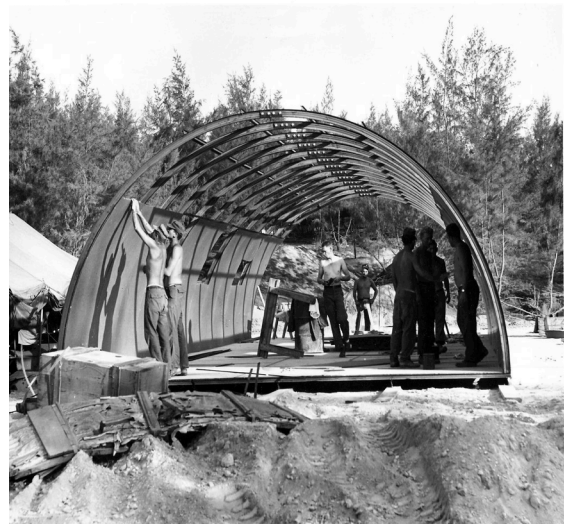
Figure 3: Construction of a Quonset Hut. Image courtesy of quonset-huts.blogspot.com.
